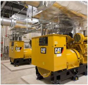
Infrastructure upgrades (generators, automation)
