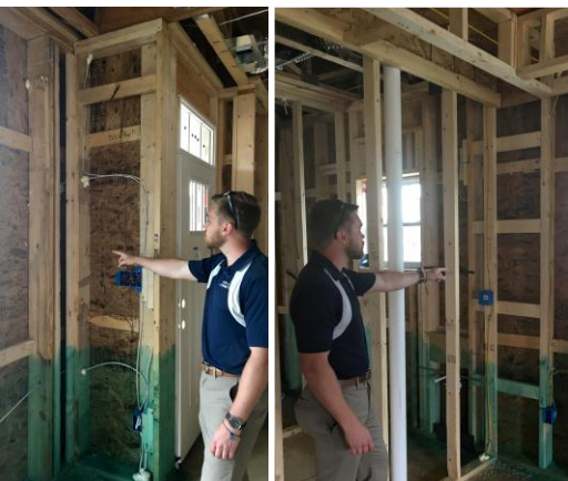
Three Stud Corner Ladder T wall
