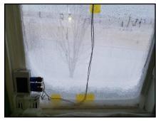
Condensation and ice buildup on existing double-pane window
