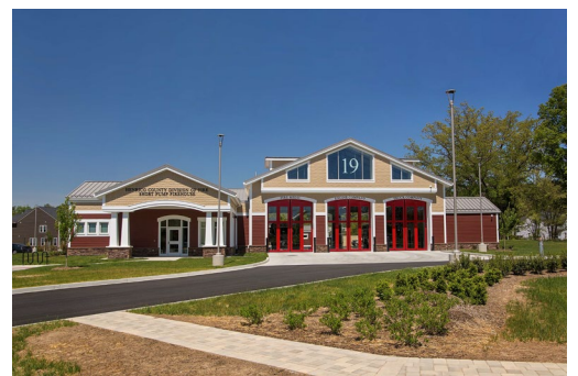
Henrico County Short Pump Firehouse 19, LEED Gold
