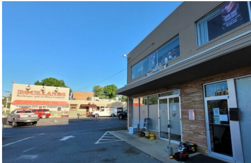
Rocklands BBQ in Arlington County is using C-PACE financing to install two solar PV systems totaling 44 kw.
