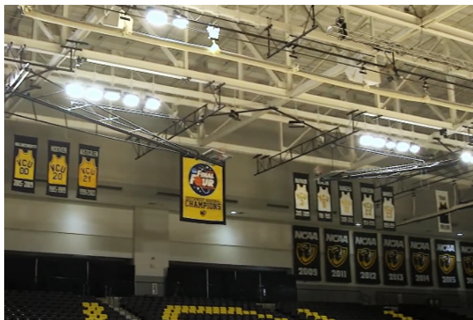
VCU used the EPC program to finance energy conservation measures in 17 buildings.
