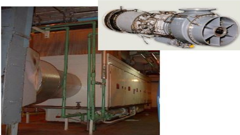
CHP plant at a brewery in London, Canada Industrial 501-KB7 Aeroderivative Gas Turbine 4.0 – 6.6 MW(e)
