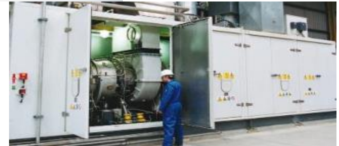
CHP plant installed in a distillery in Scotland, UK SGT-100 Industrial Gas Turbine 5.1 - 5.4 MW (e)
